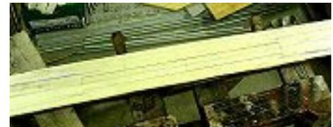
Again snap the edge centerlines. I’ve found that a quick stroke of the pull saw across the end at the level line makes a great notch to hook the chalkline into when repeatedly snapping these lines.
